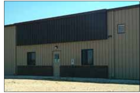
Town of Brillion Municipal Building
