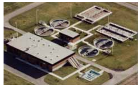
City of Brillion Waste Water Treatment Facility
