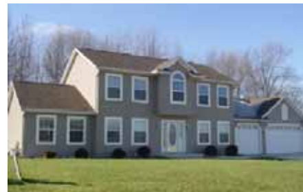
New Neighborhood home in a City of Brillion subdivision.
