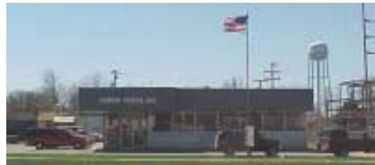
8 S Zander Press Inc. - Service 425 W. Ryan Street
